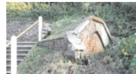
Cathedral Well Head at St James Park Station
